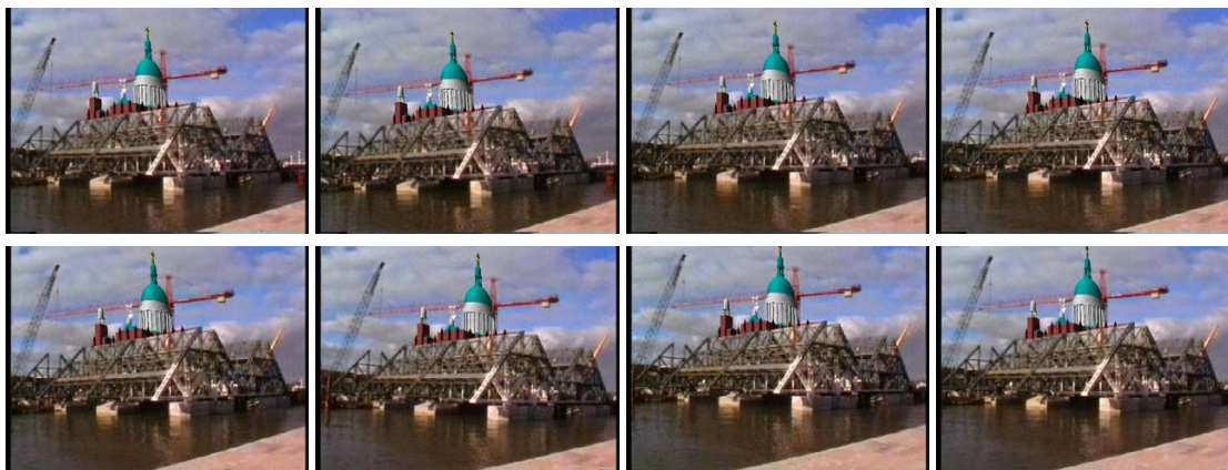
Figure C.6: Virtual tower on an outdoor construction site.
